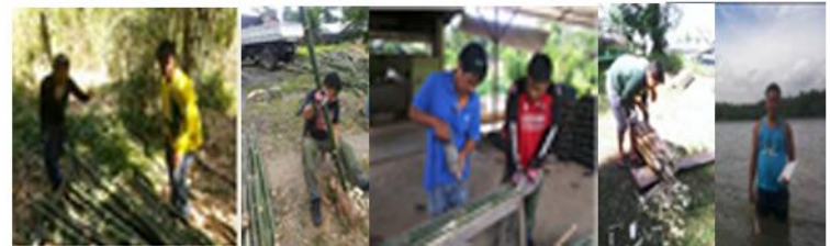
Figure 3: Construction of bamboo wave attenuators.
